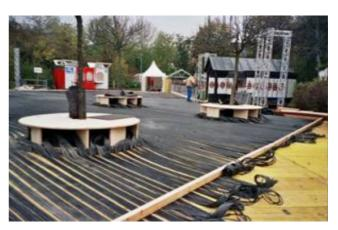
Alternatively, we can offer ice mats EPDM (roll out), in white or in black (standard version). The white mats are better during the process of Ice making because they refelct of course much better the sun You are able to make the Ice a lost faster. In operation, white mats have compared with normal black rubber no advantages.
